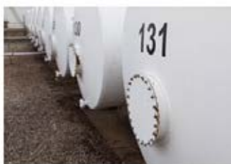
Guidance Note 57: Confined Space Entry
