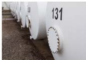
Guidance Note 57: Confined Space Entry
